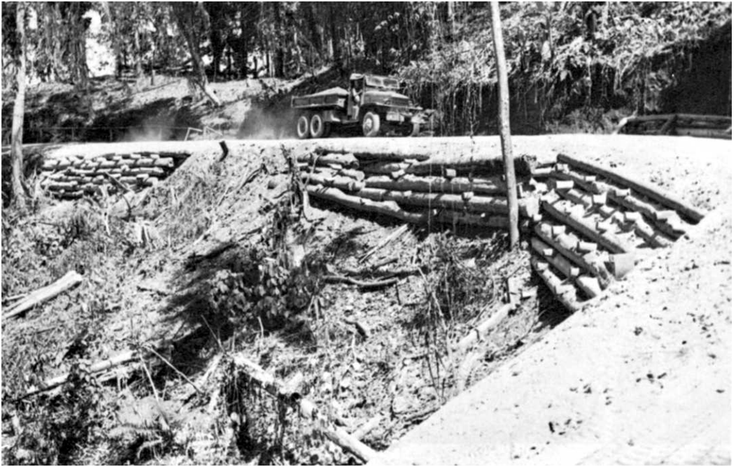
SUPPLY ROAD ON BOUGAINVILLE built by Army engineers. Note how coconut logs are used to support steep bank and underside of road.
